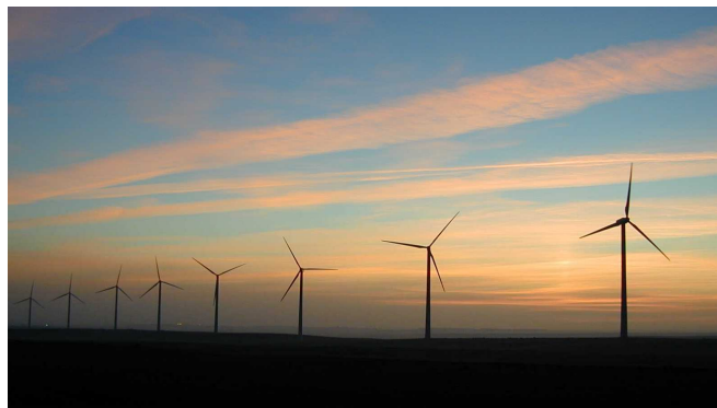
Figure 1-1: Wind turbines in Spain.
