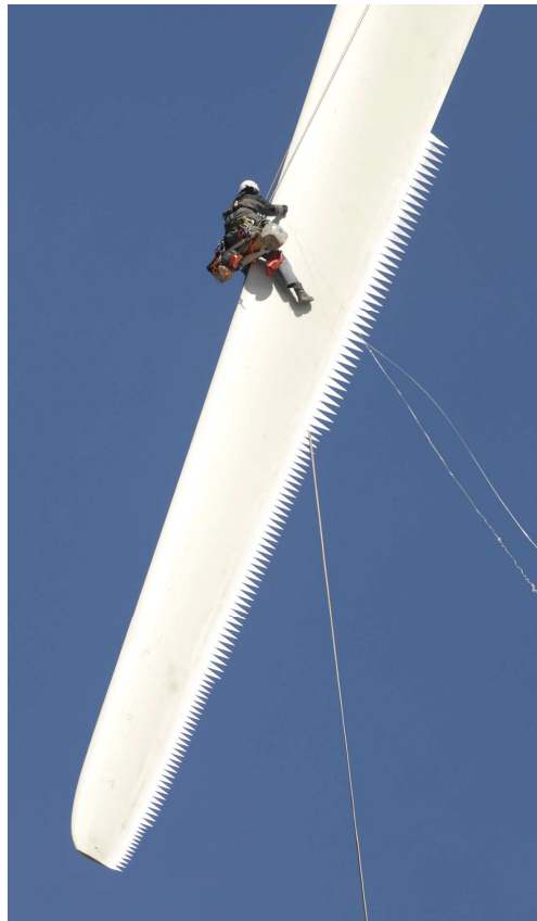
Figure 8-2: Climber removing trips from serrated blade.
